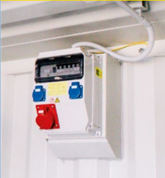
Distribution box with integrated sockets
